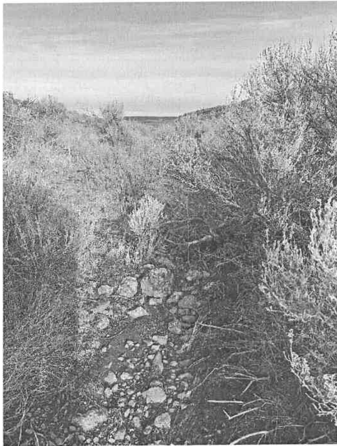
Photo 3. Evidence of storm water runoff.
